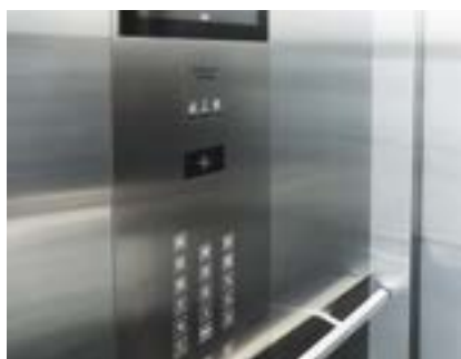
Card reader in Car Operating Panel (COP)
